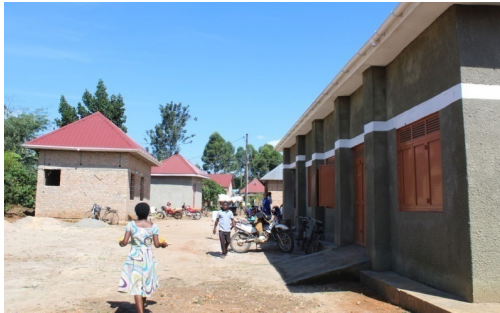
Current Structure of Kitasiba cooperative factory
