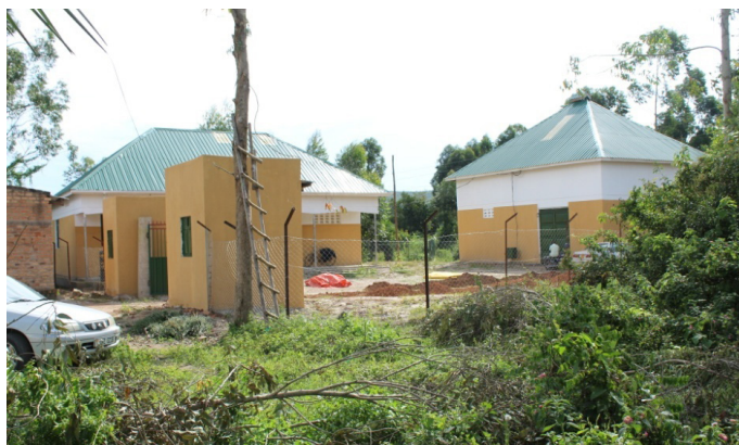
The current Lwanda farmers Coffee Factory structures which include; coffee husk chamber, an office block, a produce store, Askri shelter, kiosk, an improved pit latrine, and a huller shelter.
