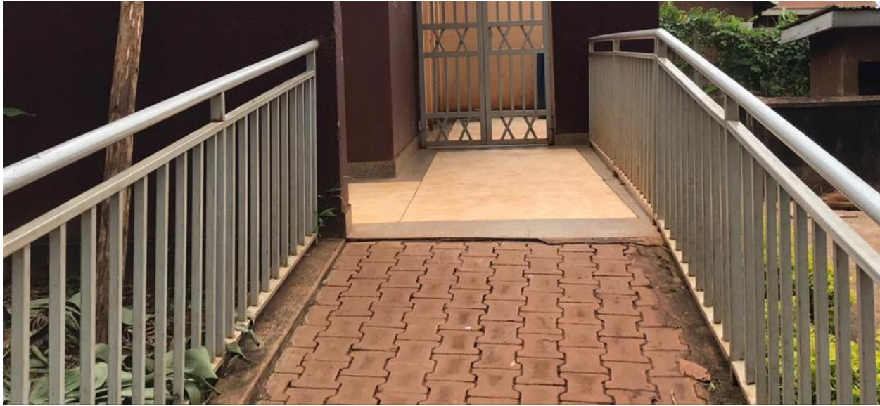
A significant number school facilities have design of a ramp to cater for disabled children
