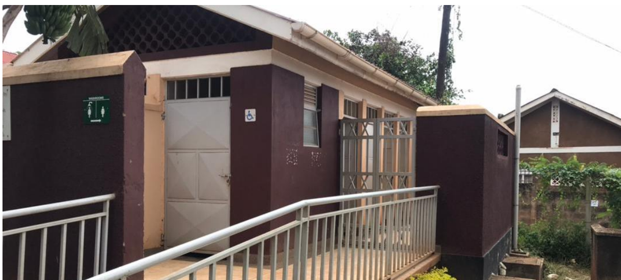
Sample toilet facility at St Paul Banda Primary School
