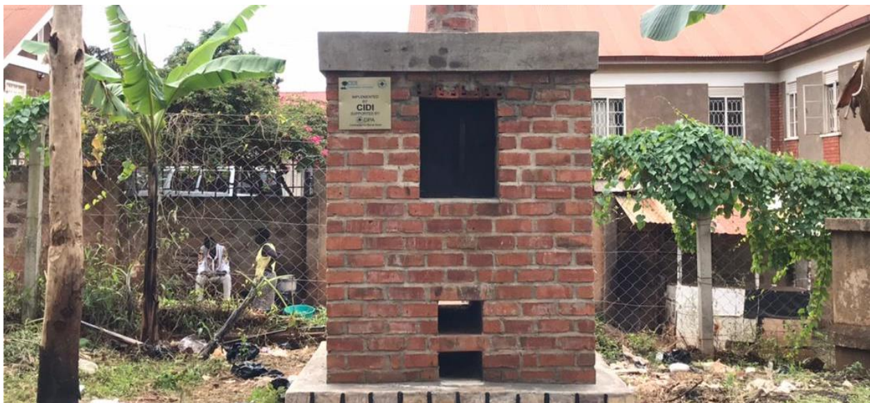
Sample incinerator in one of the schools
