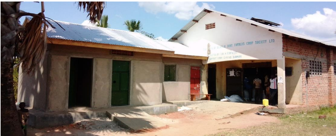
Above is the current face of OJOFACOS store with new annex for community seed bank
