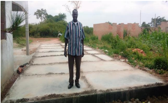
The 15Mx5M drying slab under construction at AAMCOS farmer cooperative.
