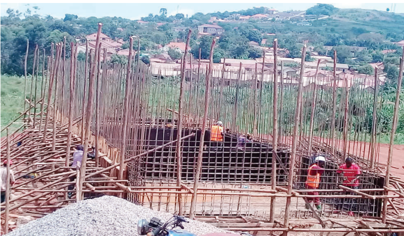
Construction of stabilization reactor for the mini treatment plant
