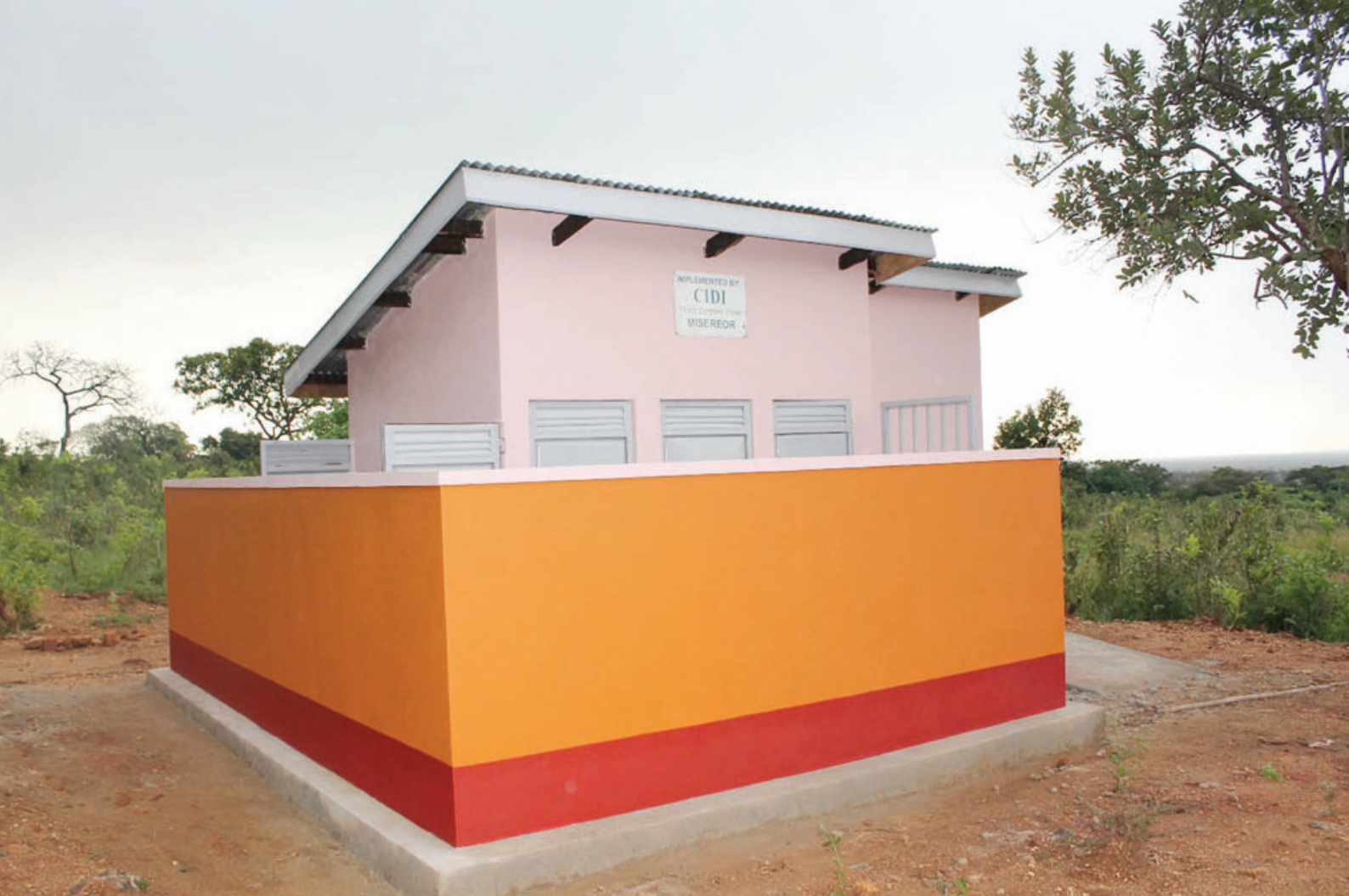
Figure 2: 7 stance drainable VIP latrine constructed in Amedek Health Center II, Napak
