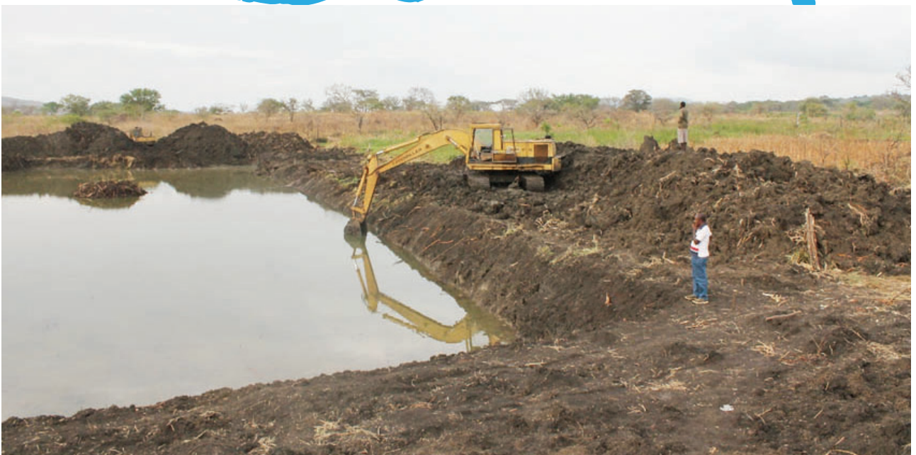
Construction of Narotol valley dam in Iriiri sub county, Napak
