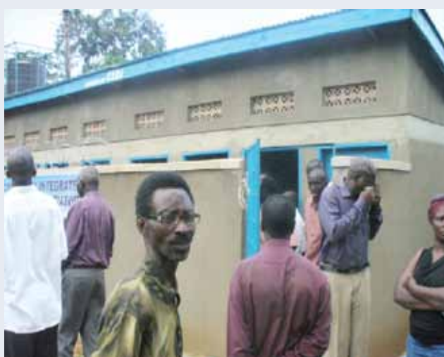
A public waterborne toilet that was established in Kabowa Parish.
