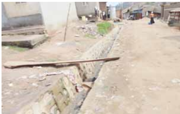
Construction of Drainage channels
