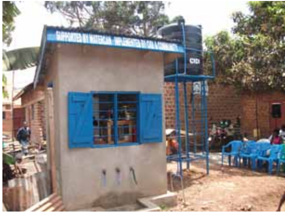
Construction of Water Kiosks
