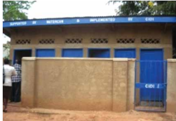
Completed public VIP Toilets
