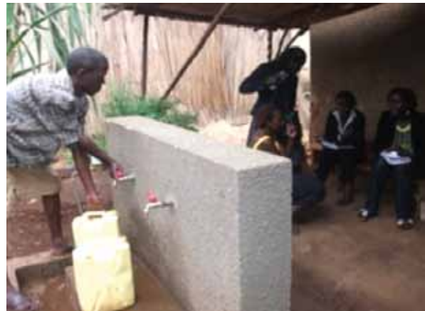
Completed public water stand pipe.
