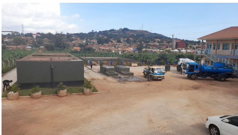
The CIDI established Fecal Sludge treatment plant in Kabojja
