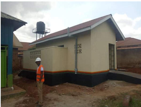
One of the completed Waterborne toilet in Lubaga
