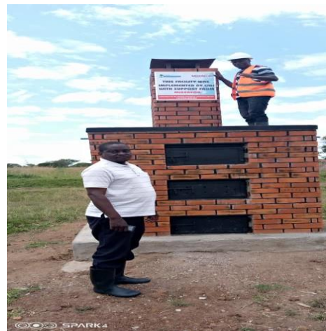
Completion of an incinerator construction.
