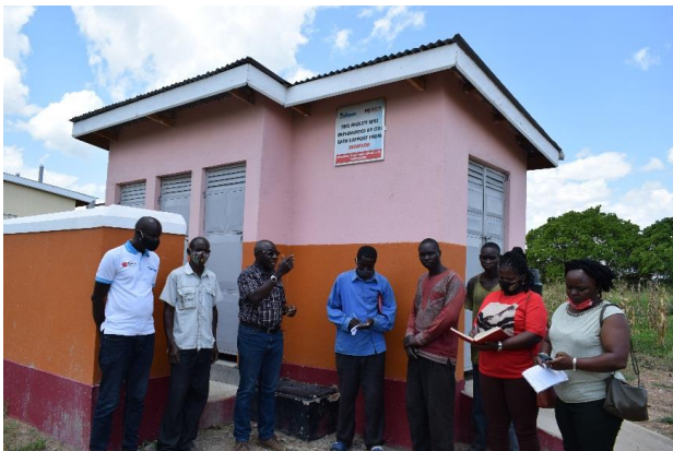
Photo showing Palam primary School Drainable VIP latrine constructed by CIDI
