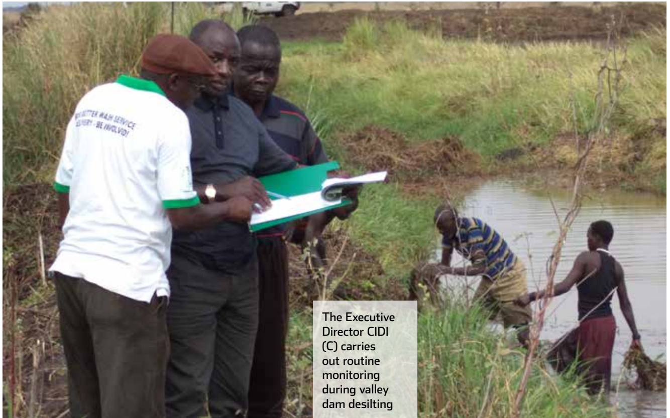
Desilting of Kalojut dam in Apeitolim Sub-county.
