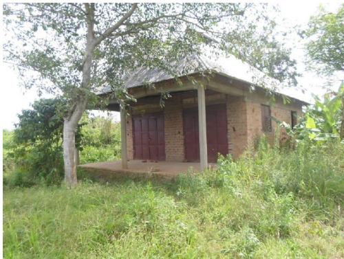
Kitasiba cooperative maize store in 2017 before upgrade using ACDP funding
