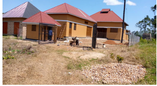
Current Kasasa Cooperative Factory, with equipped offices, Produce store, Coffee huller shelter, Askari shelter and Kiosk (Picture taken in June 2021)
