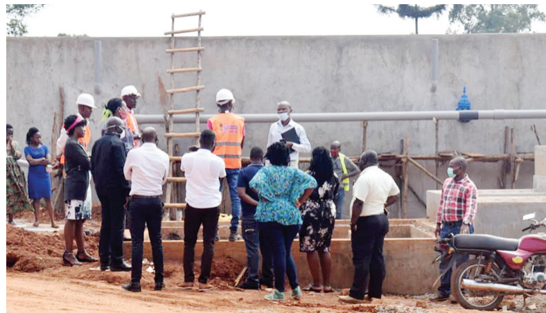
CIDI Senior Management Team and staff during the monitoring and inspection of Mini FST plant under construction in Kabojja Rubaga division.
