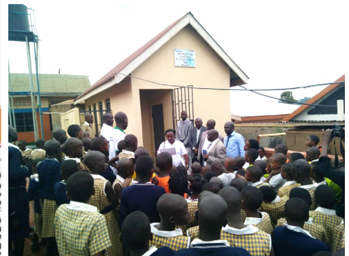
CIDI Head of WASH department at the official hand over of the newly constructed water borne toilet for Namungoona Junior school in Lubaga Division.
