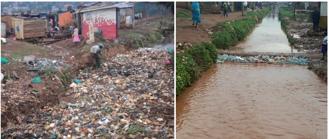
Drains full of waste gets cleaned and plastic bottles get collected for recycling. After cleaning the drains, small bridges are built with recycled bottle.
